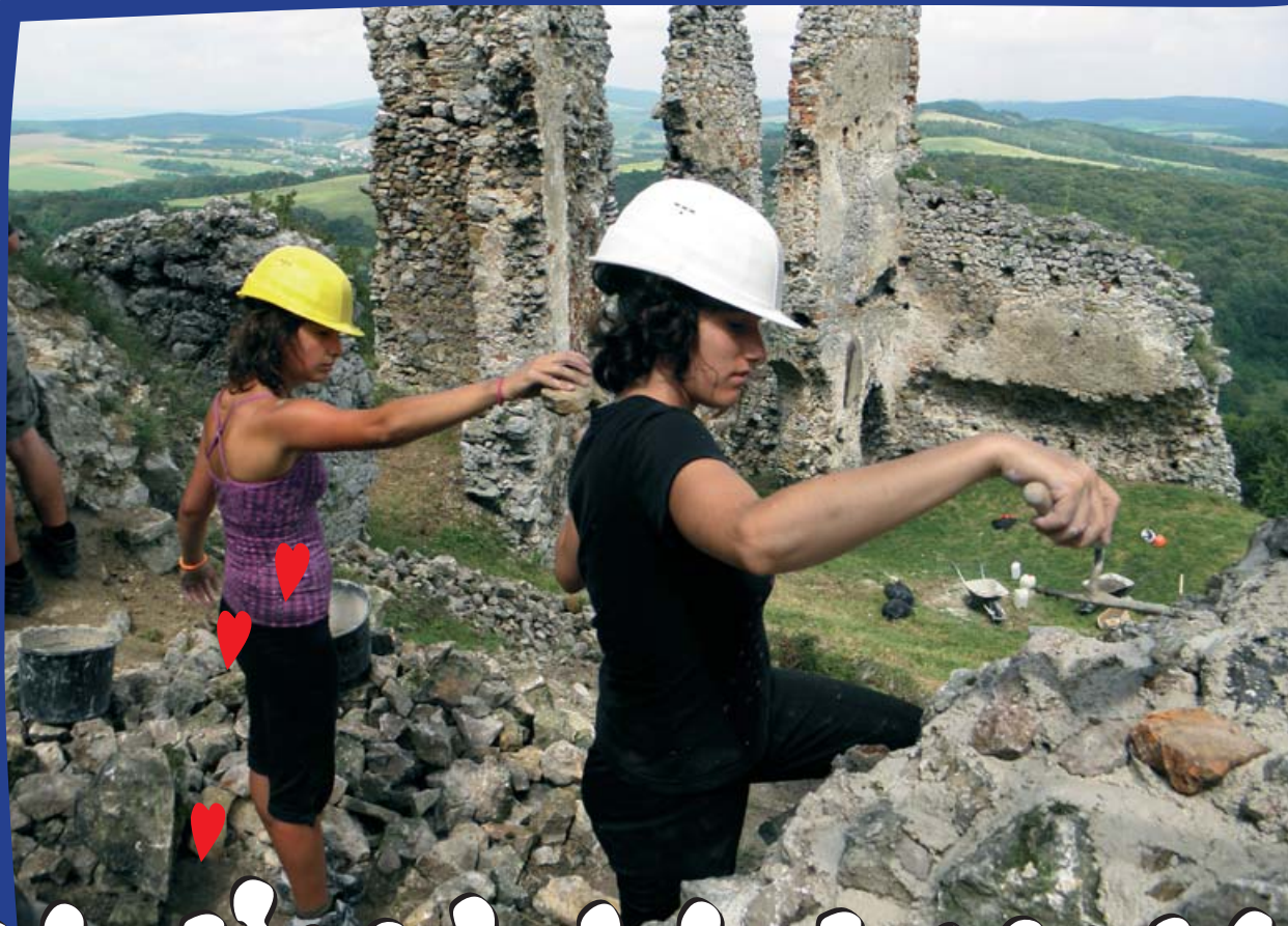
Volunteers helping with the renovation of Brekov castle in Zemplin region
